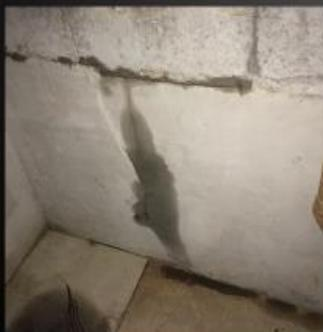
Leaking and water movement due to missing waterproofing on back side of wall
